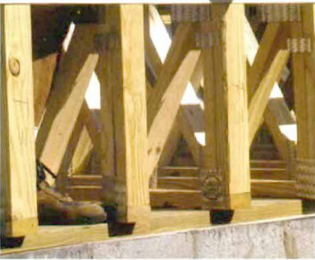
A permanent ledger connects the trusses. Once a 16-ft. row of trusses is nailed down, 2x4 ledgers can be fastened to the notches provided at the ends of the trusses.
